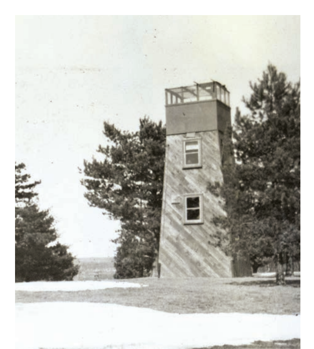
Nashawtuc Hill Fire Tower.
