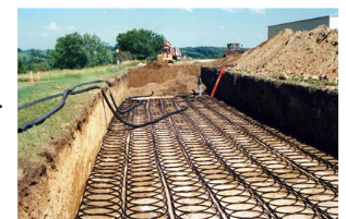
Installation of horizontal ground loop GHP. Source: www.carolinacounty.com
